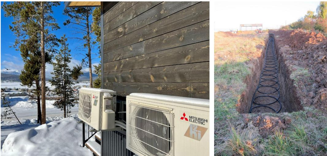
Left: Air-source heat pumps in situ (image courtesy of Joe Smyth). Right: A Slinky-style ground-source heat pump ground array (image courtesy of David Brooke). Images reprinted with permission.
